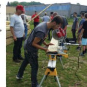
Chase Nanez '19, Ice Age Trail Boardwalk construction.
