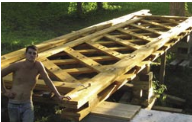
A timber side truss is laying on it’s side on the concrete footings in preparation for assembling the bridge. Raising the assembled 3,000 pound 32’ long truss was a community affair on a Saturday morning.
