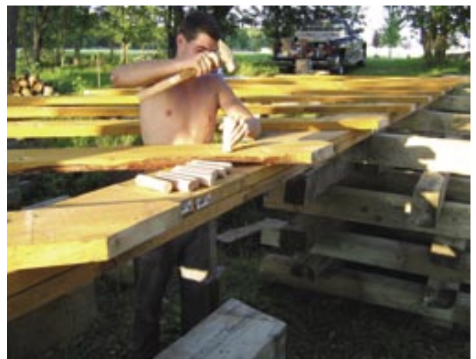
A student drives a peg into one of the trusses for the covered bridge.
